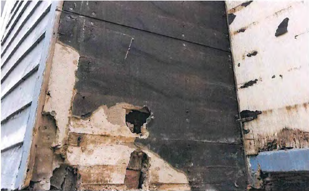
Photo 1- Gypsum Sheathing and black felt weather barrier.
