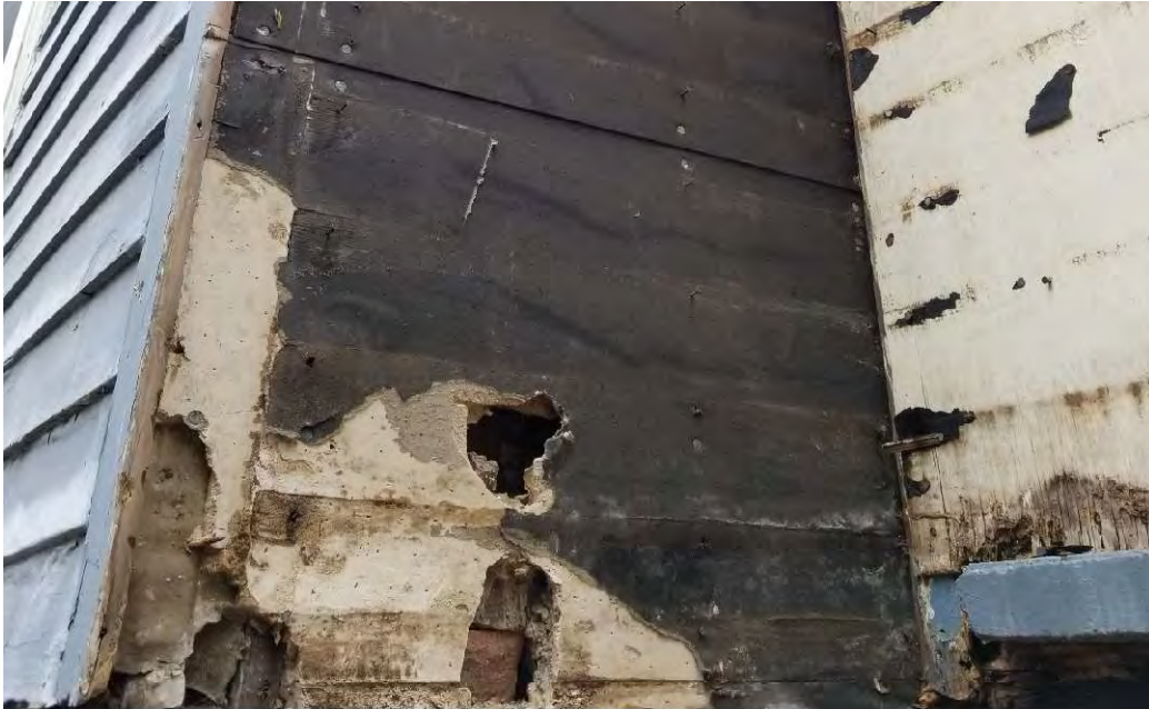
Photo 1- Gypsum Sheathing and black felt weather barrier.
